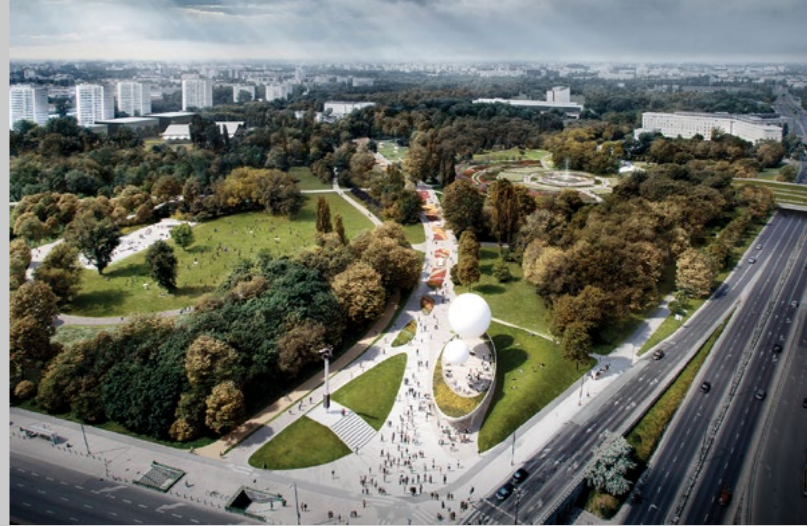
Aerial view_Park entrance_Pole Mokotowskie Park Revitalization
