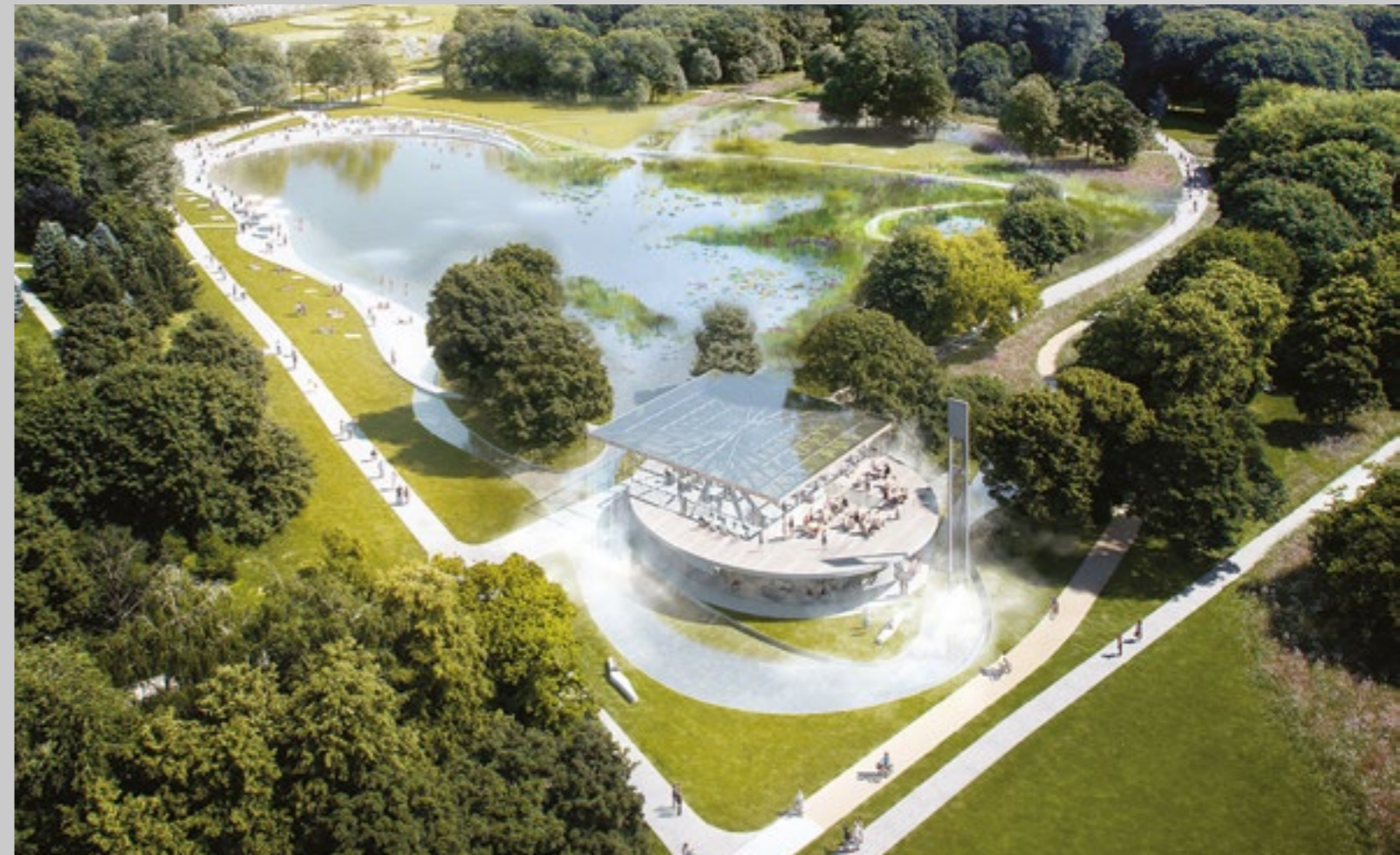
Aerial view_central lake naturalization_Pole Mokotowskie Park Revitalization
